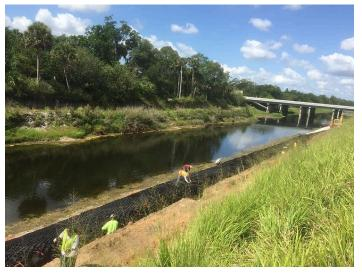
non-woven fabric, BaseCaps on top of 1/2" rebar, and tendons. This innovative approach aimed to stabilize the waterway banks, prevent further erosion, and protect the local environment.
